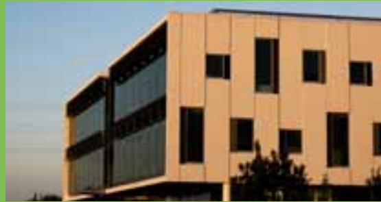
Ford Building, Highbrook Business Park Auckland
