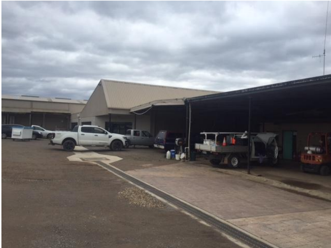
Rear Awning (linking showrooms and undercover weighbridge)
