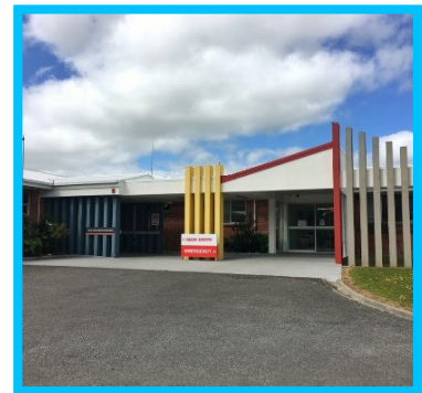
King Island District Hospital
